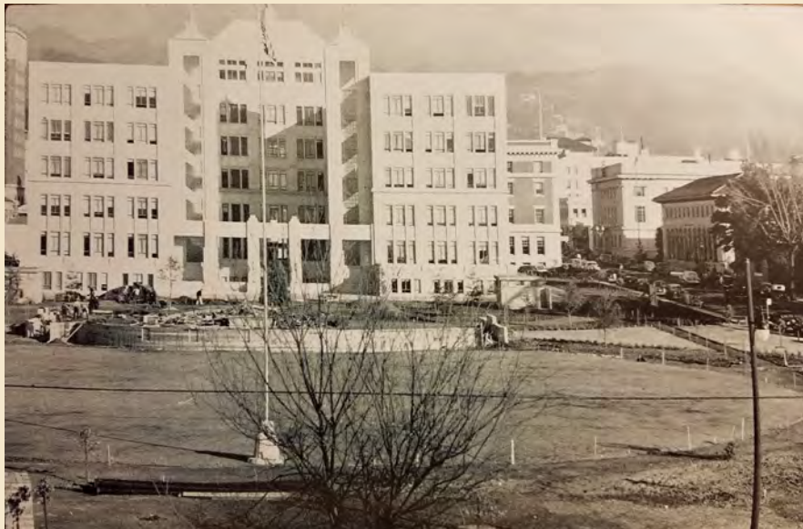
Figure 4.31 Park under construction, circa 1941. Source: Berkeley Civic Affairs , Berkeley History Collection, Berkeley Public Library.
